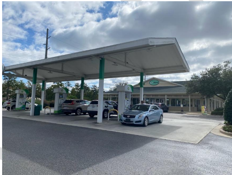
Figure 218-2. Convenience store canopy with roof form that resembles principal structure
